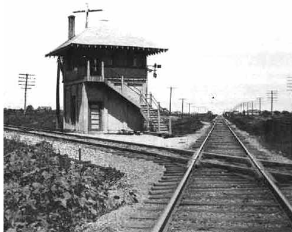
The Cotton Belt (heading to Commerce, Texas) and the Katy (heading to Greenville, Texas) cross in Hunt County Texas., in a crossover known as “Diamond.”
